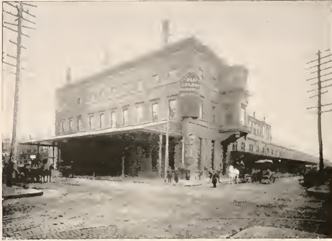
STATION OF OLD COLONY RAILROAD — MAIN DIVISION.
